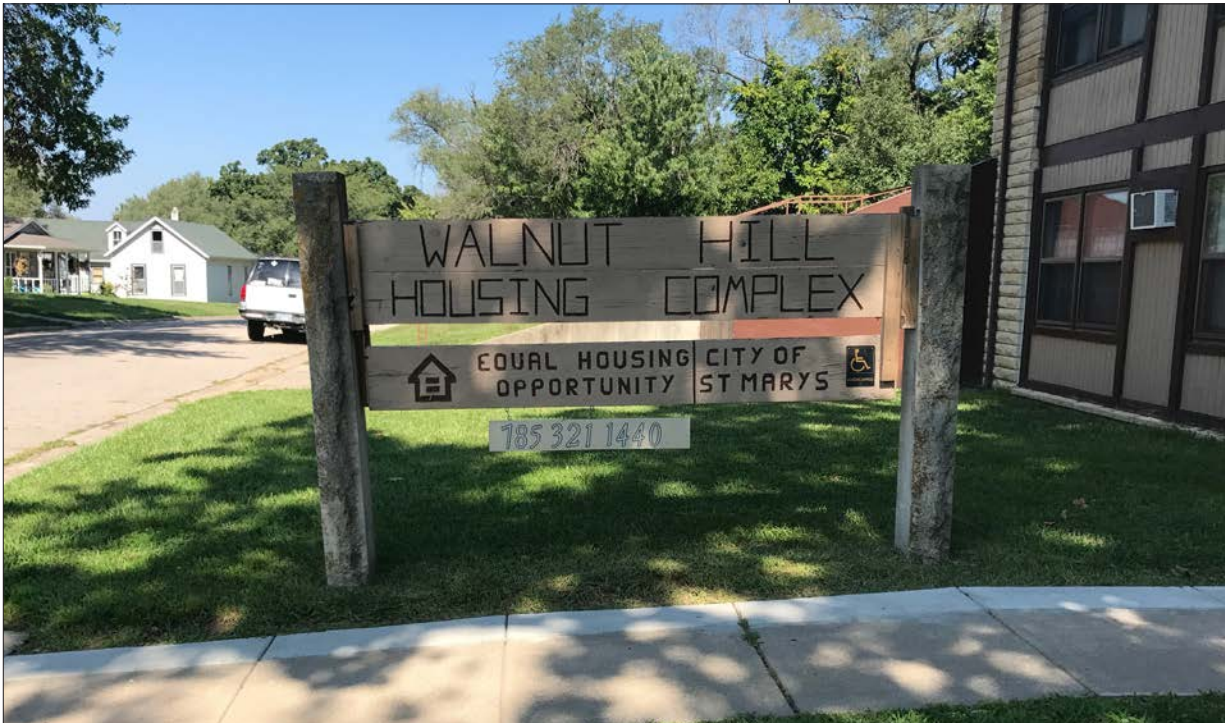
New gutters and windows are among the upgrades needed at Walnut Hill, a St. Marys, Kan., complex partially built in the 1970s.
