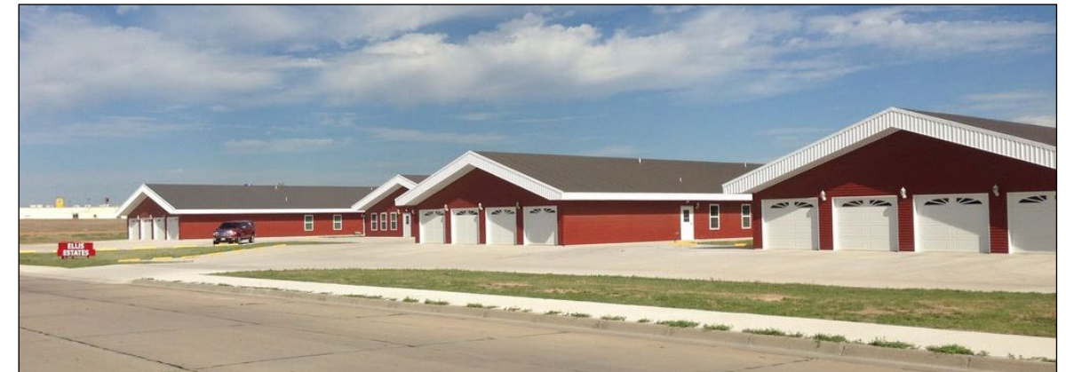
Ellis County Estates, which were funded by Farmers & Merchants Bank, include such amenities as garage access for residents.
